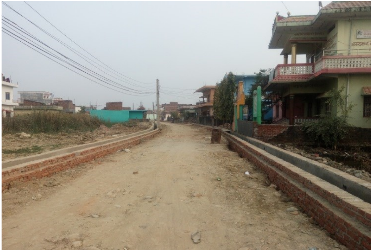
Brick Masonry Work at Shahid Path, Siddharthanagar
